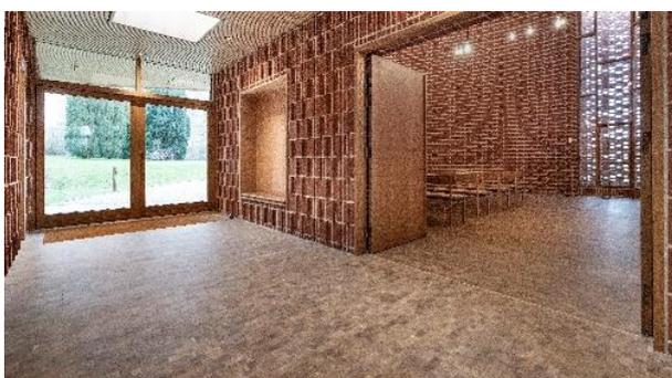
Figure 7: End Grain Floor
